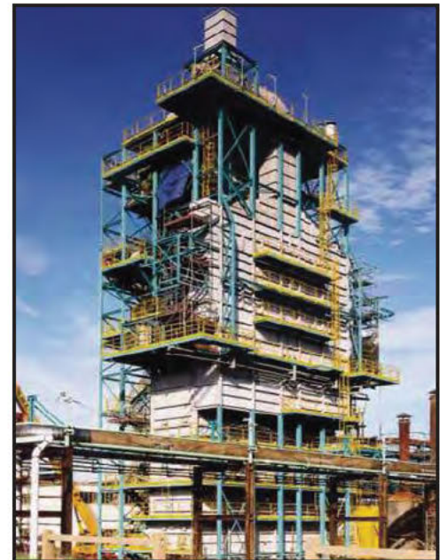
Ethylene Cracker Unit
